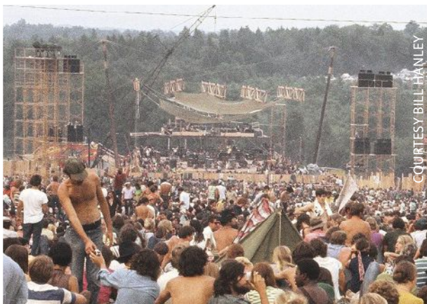
The stage view of the P.A. rig. Note the extensive use of guy wires.
