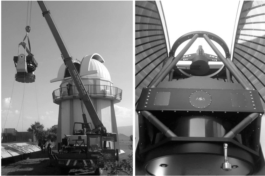
Figure 1. Left: Raising the telescope to the door of the new dome. The tube with the secondary mirror was detached and moved separately. Right: The telescope seen from the new dome.
